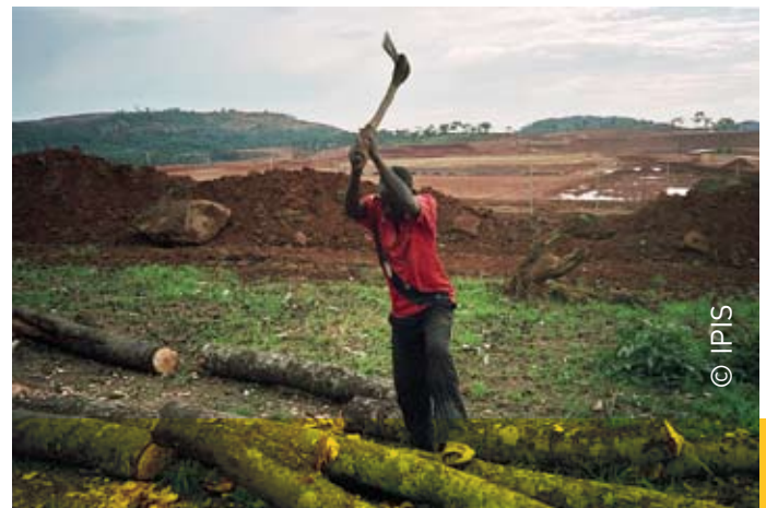
Mulumbu : man cutting a tree in front of the future site of the TFM reprocessing plant
