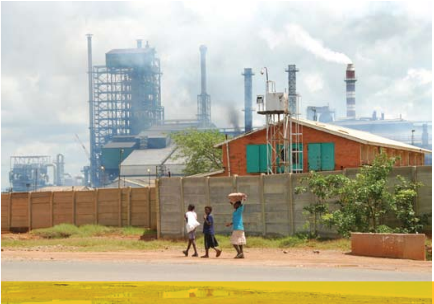
Children in Zambia passing by the EIB-financed Mufulira smelter that separates their neighbourhood from the town. Their Kankoyo neighbourhood receives all the plant's SO 2 emissions, destroying all agriculture land and making it difficult to breathe.
